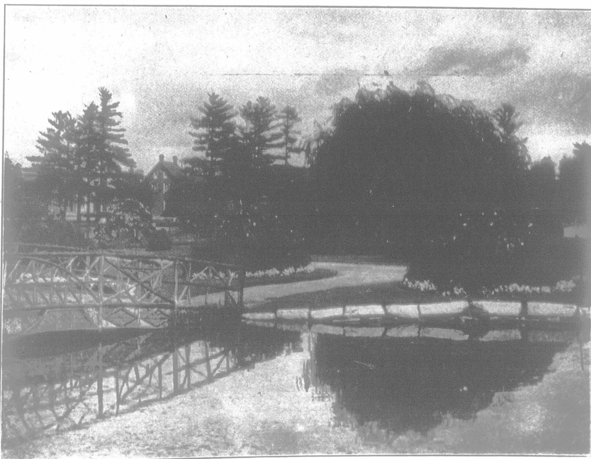
On the Rideau Canal Driveway, near Ottawa, Ont.
