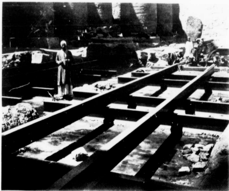
1. Hypostyle Hall; adjusting one of the columns. 2. The new foundations for the fallen columns.
