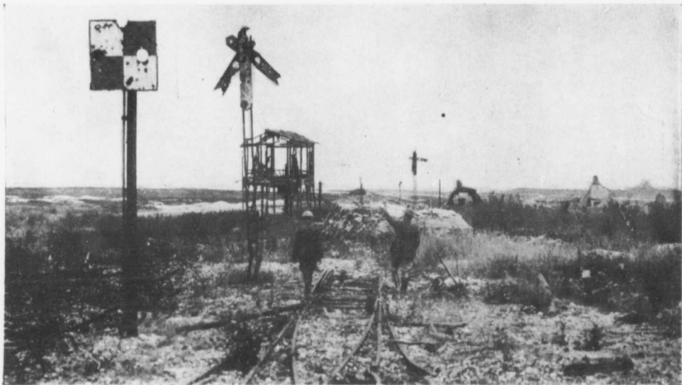
ALL THAT WAS LEFT OF A SMALL STATION NEAR LENS. THE PERMANENT WAY IS BADLY DAMAGED.
