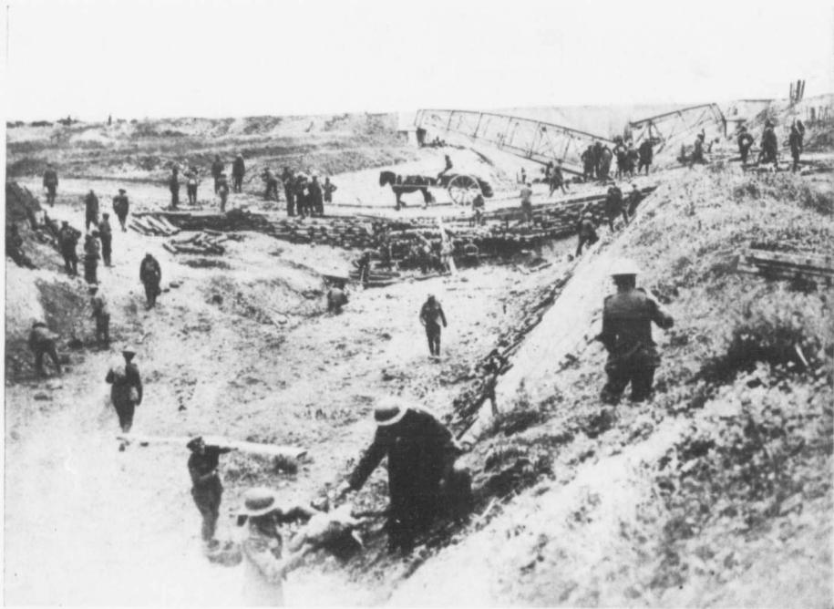
CANADIAN ENGINEERS CONSTRUCTING A BRIDGE ACROSS A RIVER ON THE ARRAS-CAMBRAI ROAD ON THEIR WAY TO CAMBRAI.
