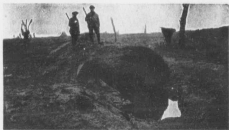
THESE CONCRETE STRONG-POSTS WERE USUALLY HALF SUNK LIKE THIS, AND THEREFORE PRESENTED A VERY SMALL TARGET.
