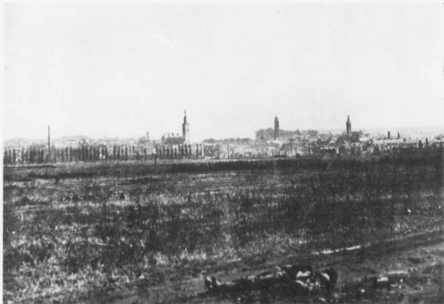
A VIEW OF CAMBRAI DURING THE ADVANCE OF THE CANADIAN ARTILLERY ON OCTOBER 1, 1918.
