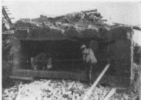
THE STRENGTH OF THESE FORMIDABLE CONCRETE DEFENCES SHOULD BE NOTED.
