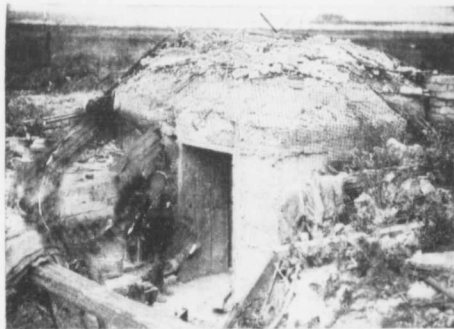
GERMAN DUG-OUT CONSTRUCTED WITH CONCRETE AND IRON GIRDERS, IN TRENCHES NEAR LENS CAPTURED BY THE CANADIANS.
