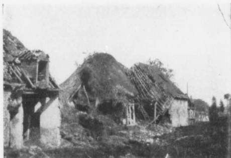
SHATTERED HOUSES IN A VILLAGE WHICH FREQUENTLY CHANGED HANDS.
