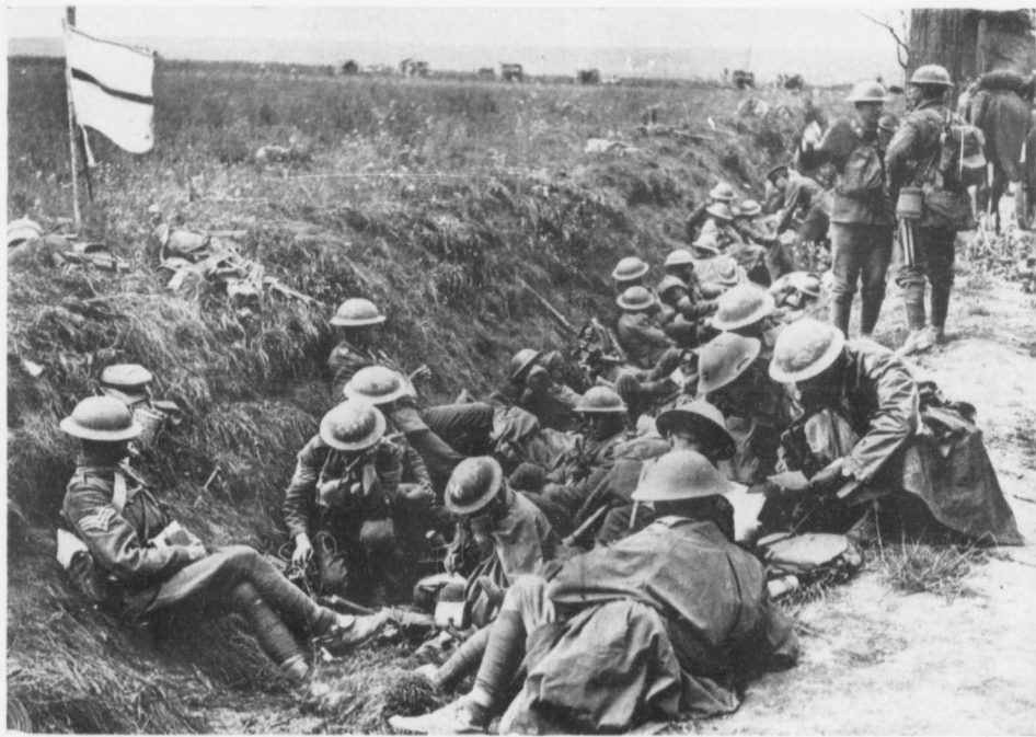
BRIGADE HEADQUARTERS DURING THE AMIENS ADVANCE.
