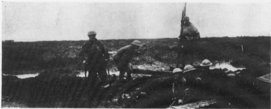
CANADIAN PIONEERS LAYING A TRACK OF DUCK-BOARDS AMONG THE MUD AND SHELL HOLES AT PASSCHENDALE OVER WHICH THE WALKING WOUNDED COULD COME OUT.
