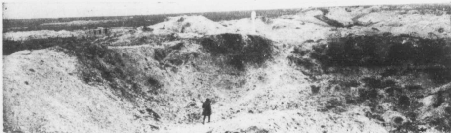
A MINE CRATER ON THE RIDGE : BEHIND IS SEEN A MEMORIAL TO FALLEN CANADIANS.
