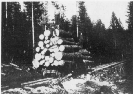
CANADIAN FORESTRY CORPS WORK IN FRANCE.
