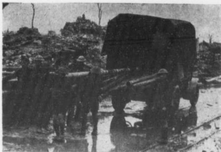
UNLOADING WATER PIPES.
