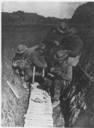
SIGNALLERS REPAIRING WIRES IN A COMMUNICATION TRENCH NEAR THE FRONT LINE.
