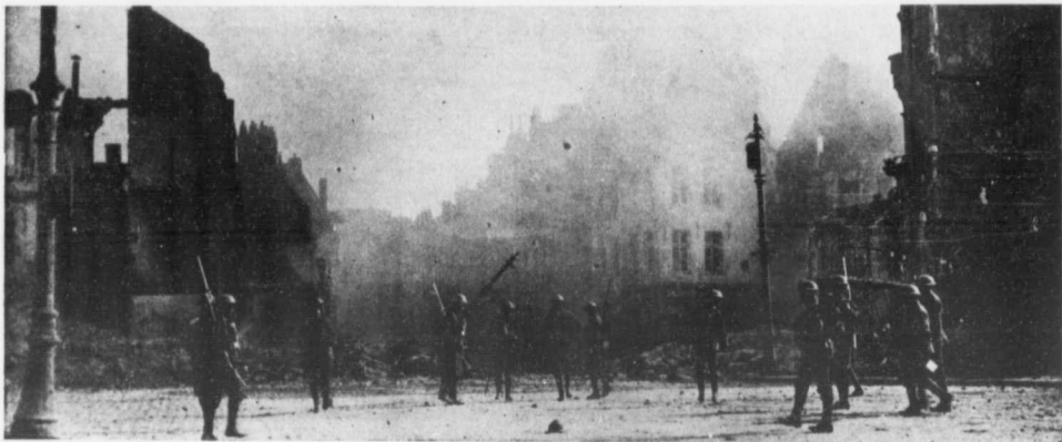
ON ENTERING CAMBRAI THE CANADIANS FOUND GREAT DAMAGE CAUSED BY GERMAN MINES AND FIRES.
