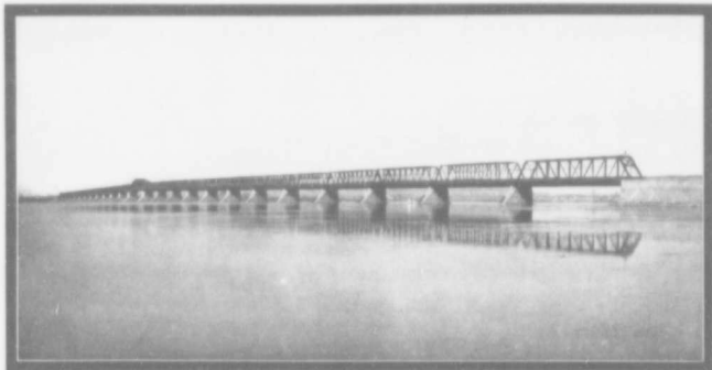
GRAND TRUNK VICTORIA JUBILEE BRIDGE OVER THE ST. LAWRENCE RIVER, MONTREAL.
