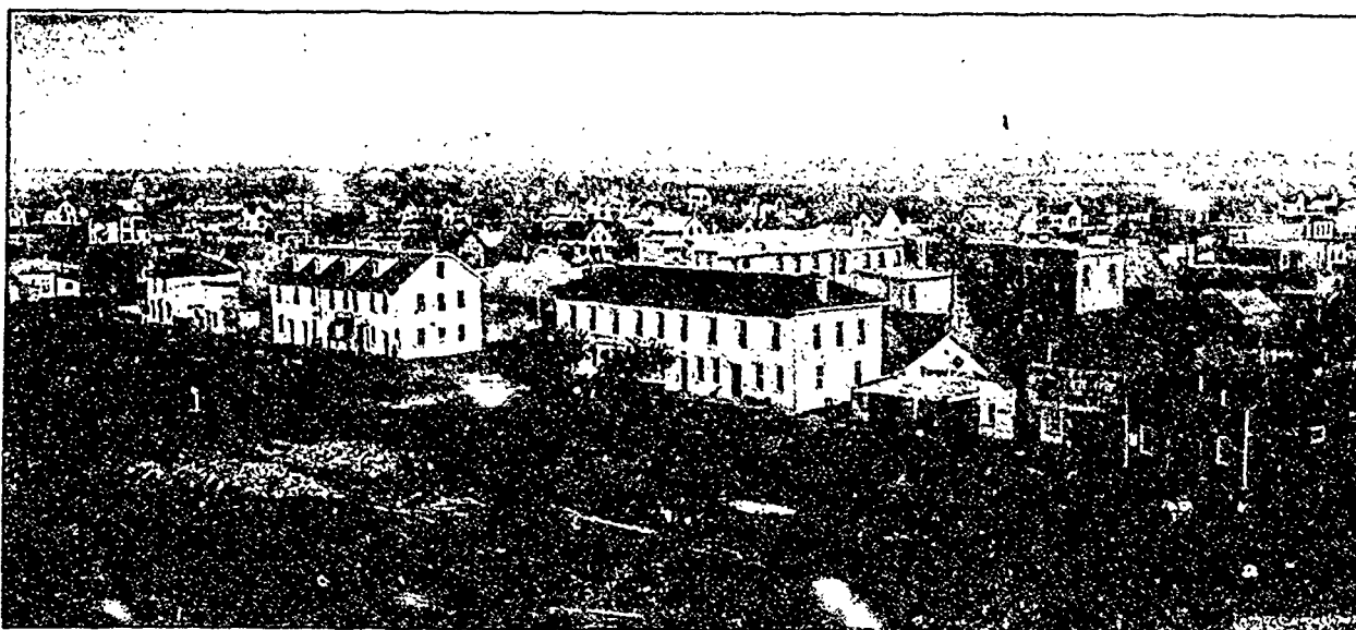
CARBERRY, MAN., LOOKING NORTHWEST FROM LYONS' ELEVATOR.
