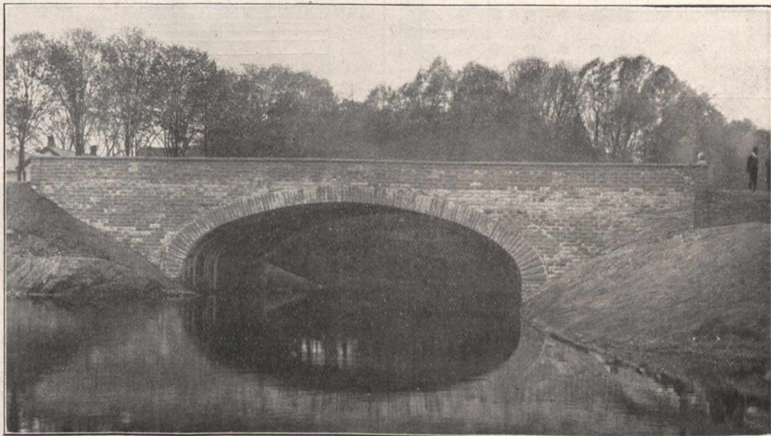
Concrete Bridge with Concrete Block Face, Union Street, Owen Sound.
