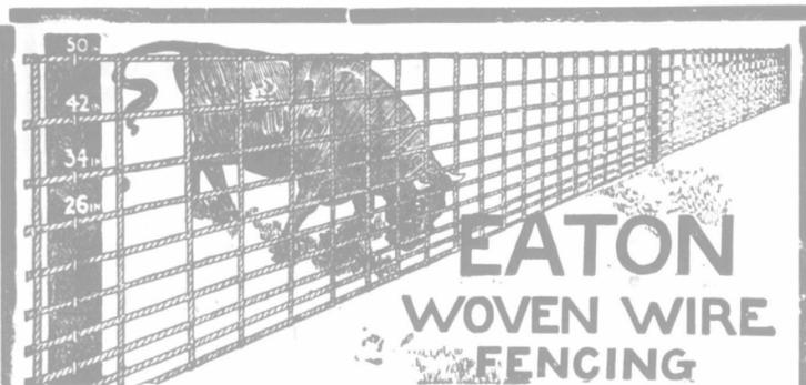
Here is a fence high enough for horses, close enough for hogs, strong enough for cattle—a splendid barnyard fence. It is made of No. 13 Galvanized Steel Wire, doubled and twisted. The stays are placed 12 inches apart, and securely interlocked to prevent slipping.
