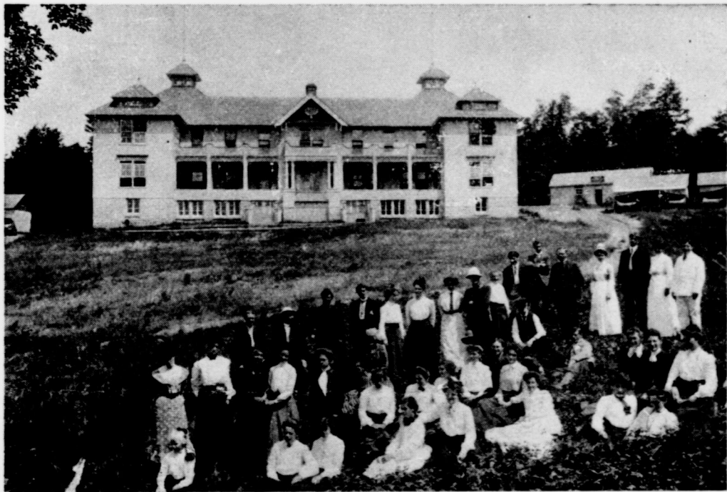
ADMINISTRATION BUILDING, MUSKOKA FREE HOSPITAL FOR CONSUMPTIVES.
