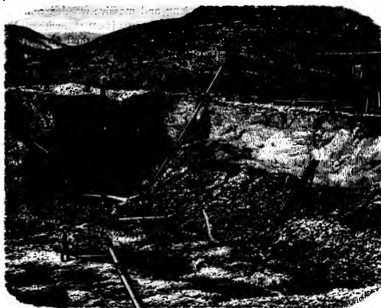
PERRY'S HYDRAULIC ELEVATOR AT WORK.
