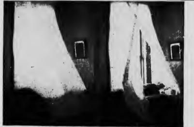
By concretely of Dc. T. S. Carcington.] Home-made Window Tent. This is made with two sheets 9 feet long by 4 feet wide. Tack to Window Casing and attach by Tape to the Floor.
