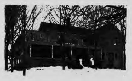
LOOMIS SANATORA M. CHARMAN COTTAGE. A REMODELTED FARMADIOLSL. THE BUILDING OF SUTTING PORCHES, INSTATUNG OF SUTARIA HEATING PLANT, TEARING DOWN PARTITIONS AND CUTTING DOWN DOORS COST \$1,200.
