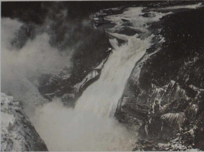
Almost twice the height of Niagara, Churchill Falls provides the energy for the largest hydro electric generator plant in the world, located underground.
