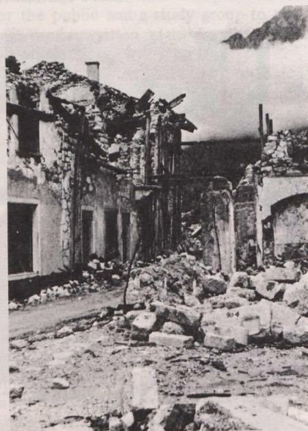
Over 1,000 people were killed and 150,000 made homeless in the earthquake.
