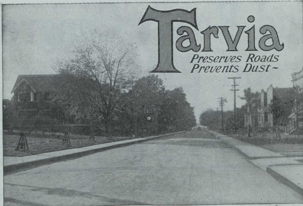
Rockland Avenue, Outremont, Quebec. Constructed by Tarvia Penetration Method.
