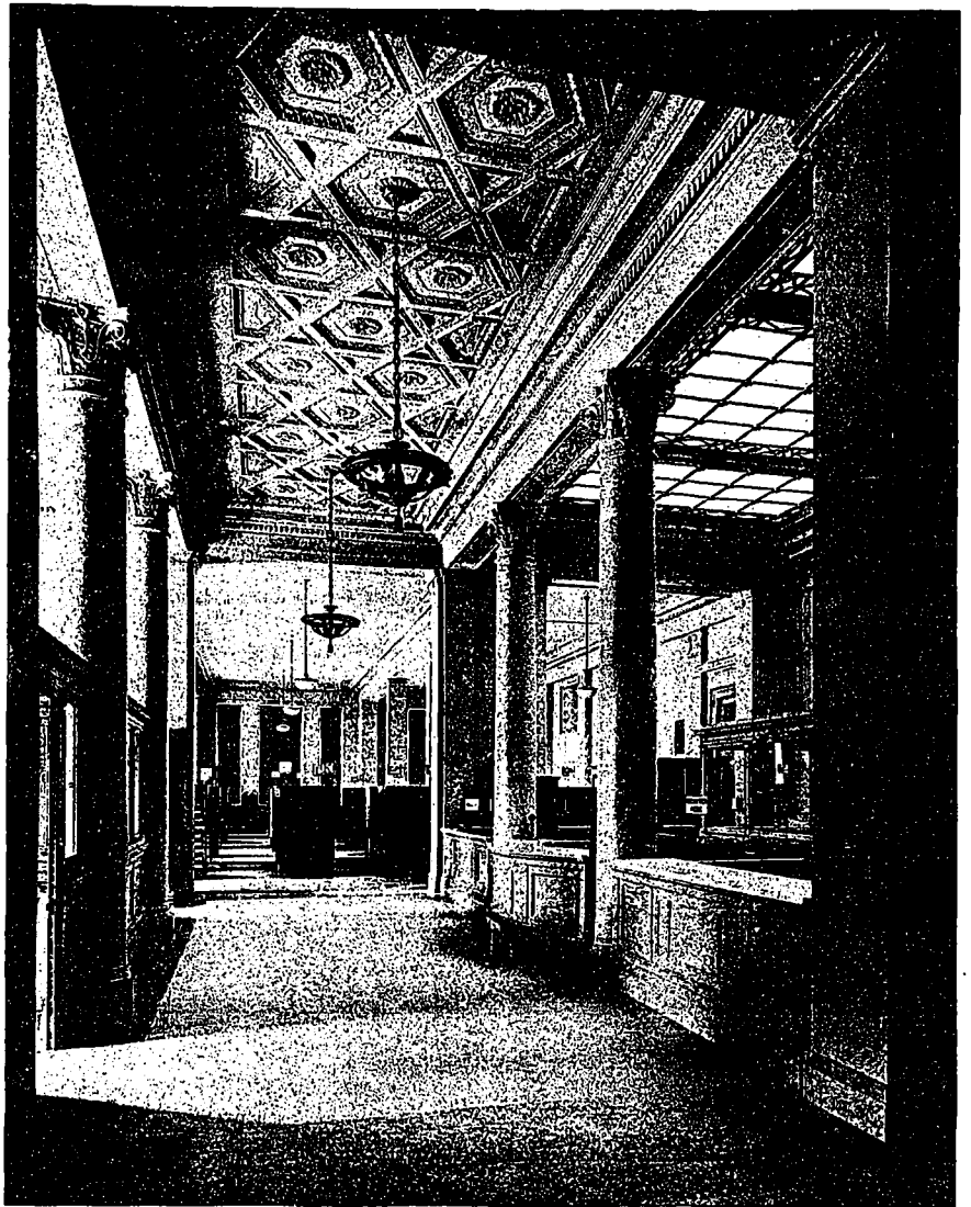
PUBLIC SPACE, REGISTRY DIVISION, REGISTRY OFFICE, TORONTO.
