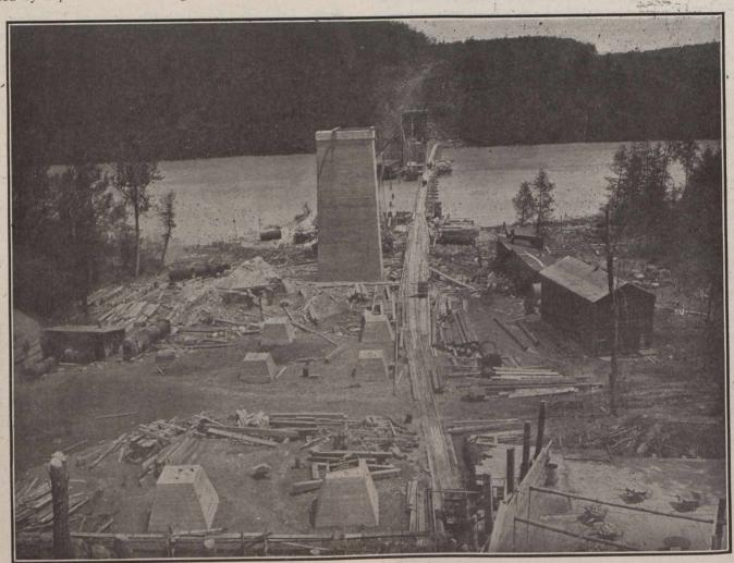
Fig. 4.-Bird's Eye View Looking East, Showing Pedestals for Steel Work, and Pier No. 4 in the Foreground.
