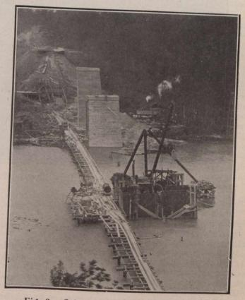
Fig. 3.-Caisson for Pier No. 2 Being Sunk.
