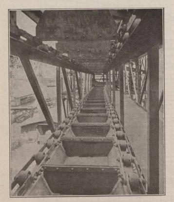
Fig. 1.—100-ton-per-hour Flight Conveyer, 360 Feet in Length, Used by the Philadelphia Rapid Transit Co.
