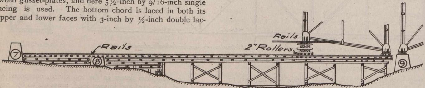
Fig. 5.—Staging Track for Moving Towers Into Place.
