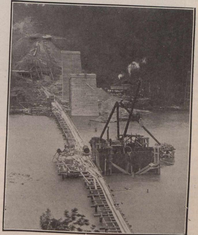
**Fig. 3.—Caisson for Pier No. 2 Being Sunk.**
