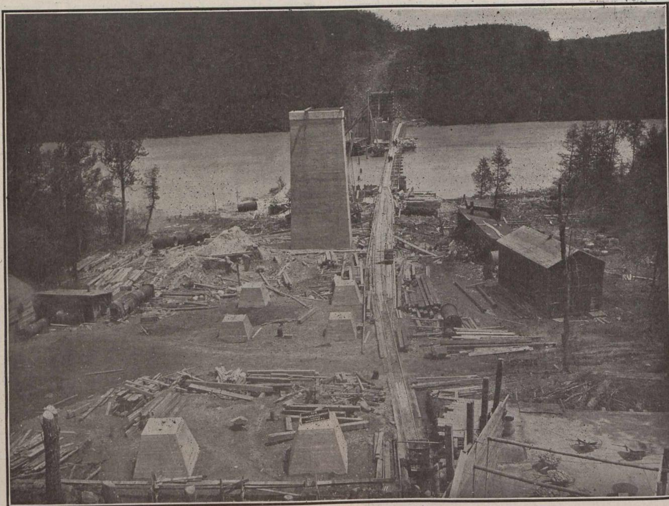
Fig. 4.—Bird's Eye View Looking East, Showing Pedestals for Steel Work, and Pier No. 4 in the Foreground.
