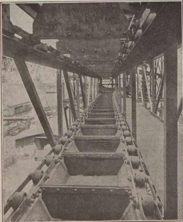
Fig. 1.—100-ton-per-hour Flight Conveyer, 360 Feet in Length, Used by the Philadelphia Rapid Transit Co.
