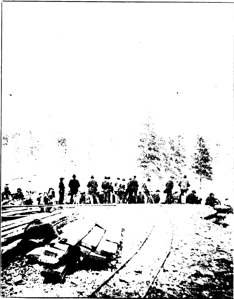
"JOE DANDY" ORE DUMP, FAIRVIEW, B.C.
