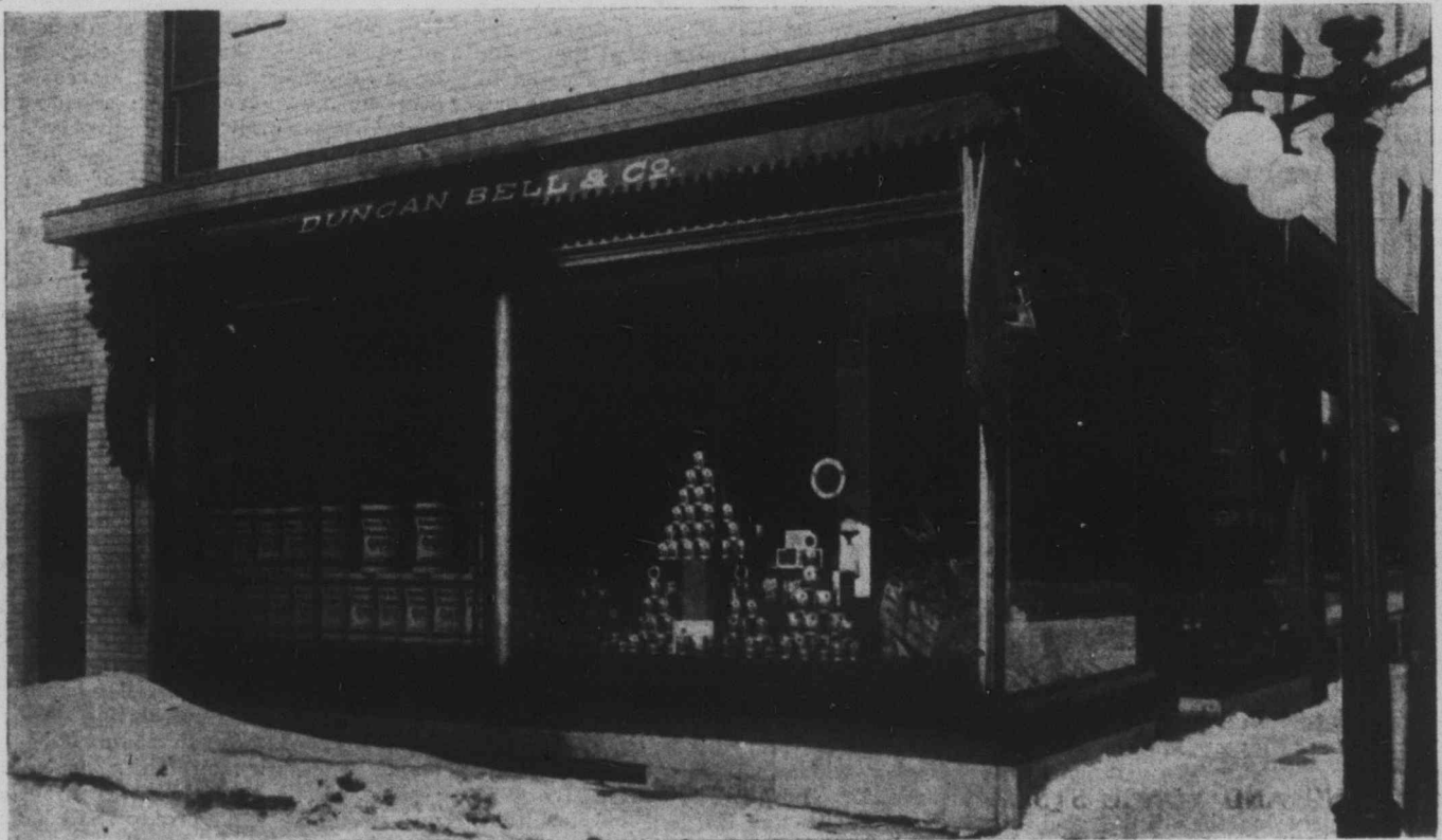
Exterior of the Duncan Bell & Co. store, Bank Street, Ottawa, showing fine display windows.
