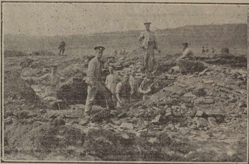
Engineers Trench Digging at Buxton.
