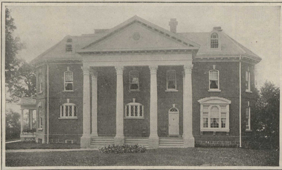
A COUNTRY HOME, REMODELLED IN GEORGIAN STYLE. This is the North Front Showing the Added Portico with Corinthian Columns.
