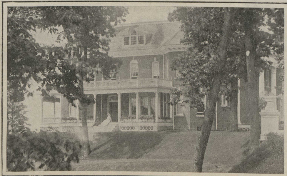
The East Front of the Same House—"Hillcrest," Port Hope.
