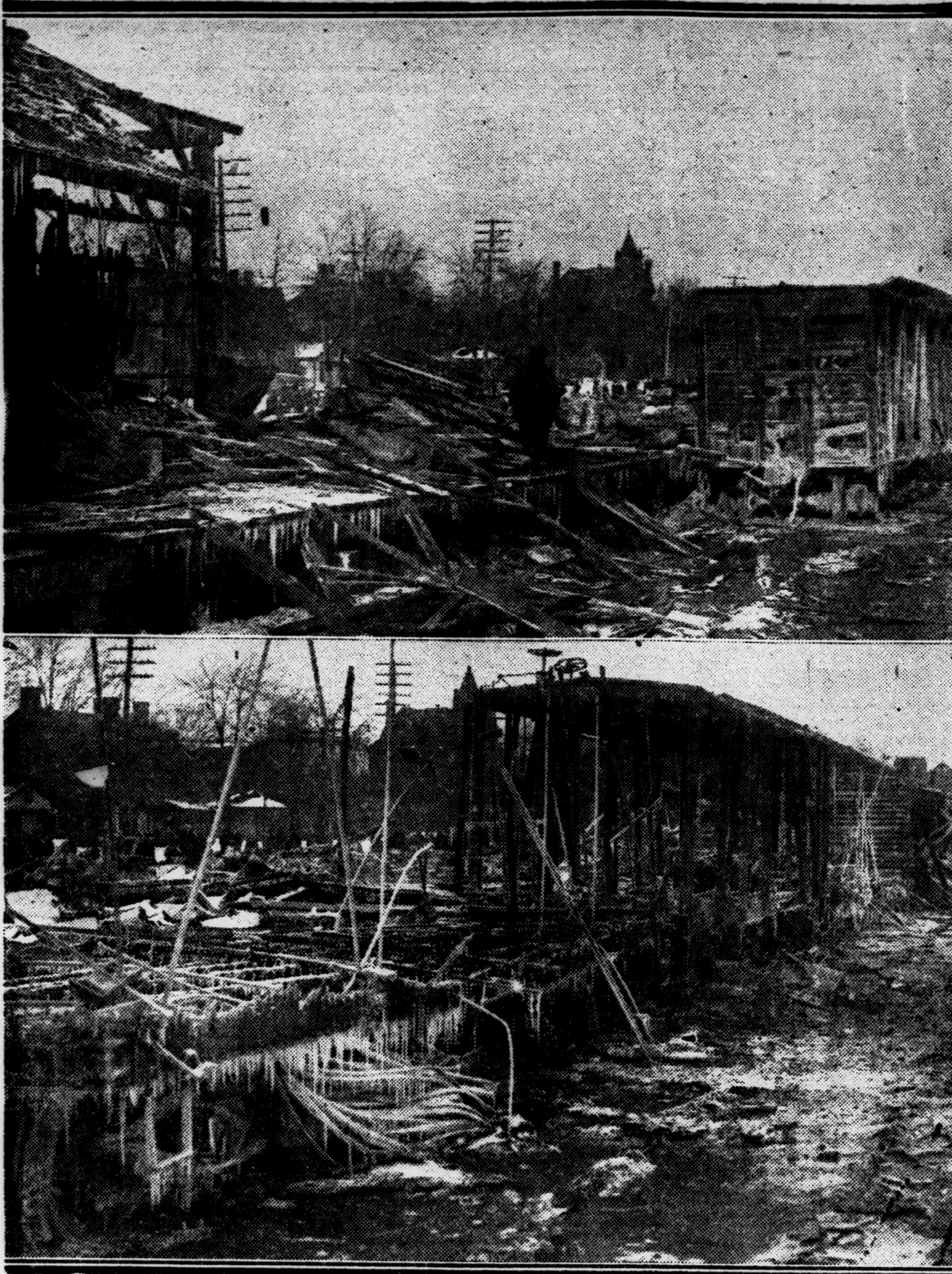
Upper picture shows Wellington street and the burned-out freight sheds. Below: Close-up view of gutted freight cars. The skeleton of one car is still intact; of the other, all that remains is the metal bed.
