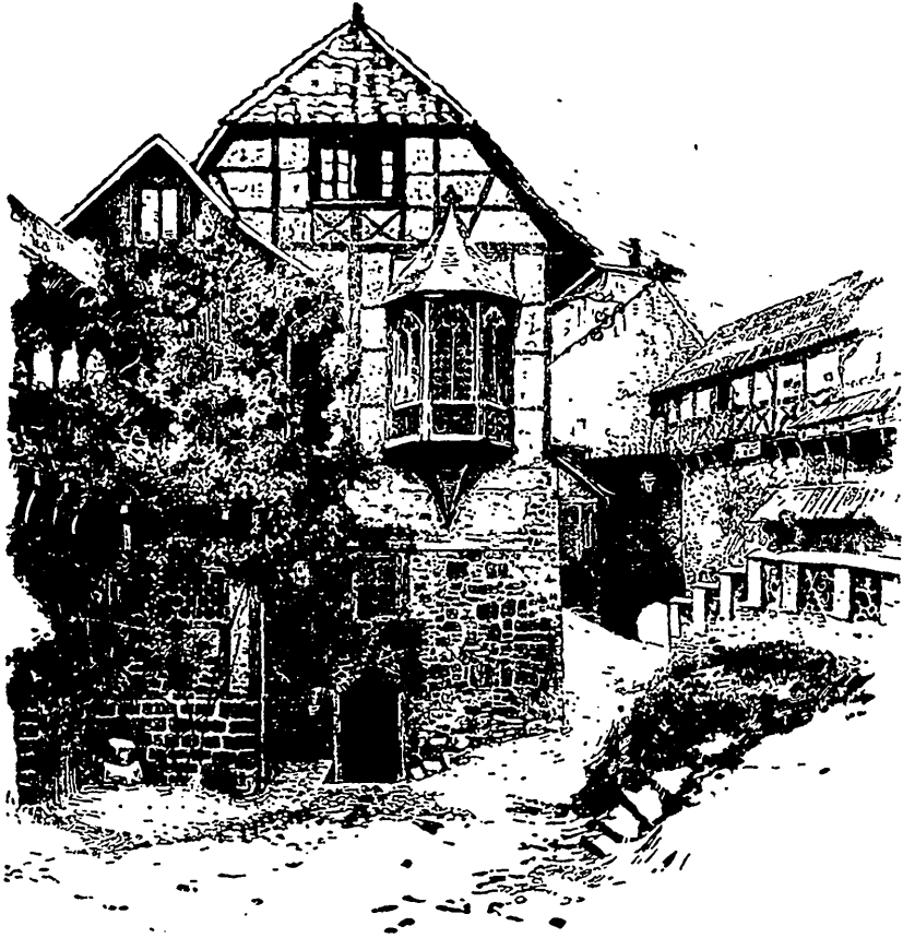
THE FIRST COURT, WARTBURG.
