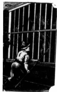
STANDING BY USE OF POLES.
