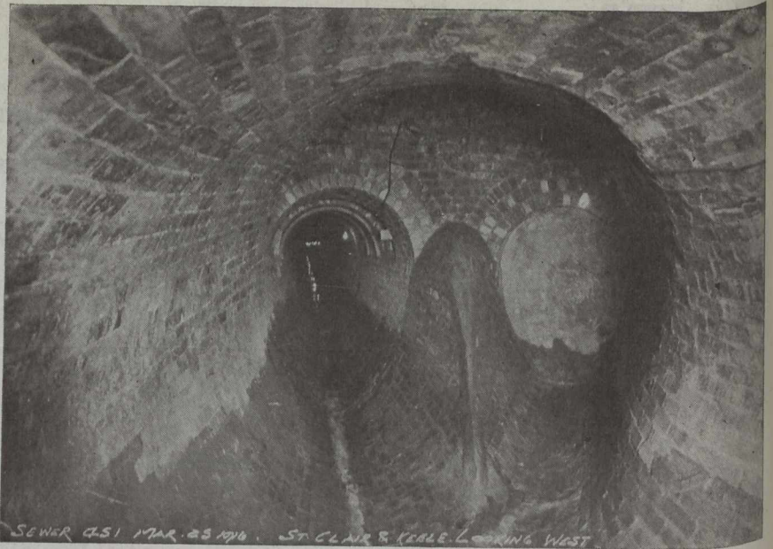
Intersections of Weston Road South Sewer with that on St. Clair Avenue.
