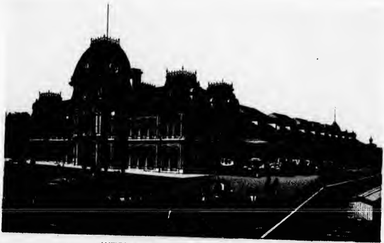
INTERCOLONIAL RAILWAY STATION.
