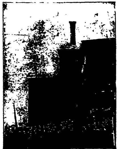
The same Chimney AFTER THE American stoker was installed.
