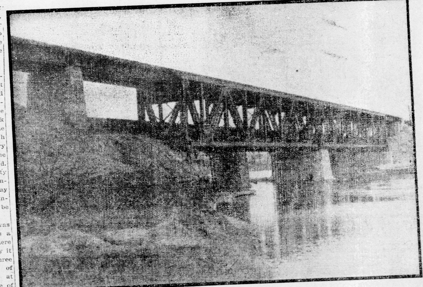
From Photo by Staff Photographer. THE GRAND TRUNK IMPROVEMENTS WEST OF LONDON—THE MAGNIFICENT NEW BRIDGE OVER THE THAMES, AT THE COVES—IMMEDIATELY TO THE REAR IS SEEN THE OLD COVE BRIDGE. THE TRACKS AT THIS POINT HAVE BEEN RAISED 30 FEET.
