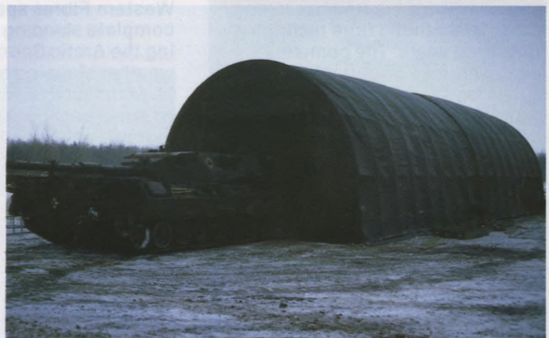
Second line insulated maintenance module for the Department of National Defence.
