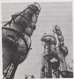
Petroleum in mist form is distilled in a "fractionating tower".
