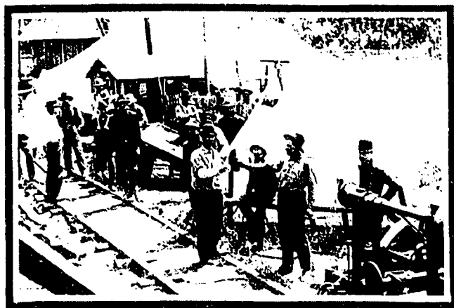
RAILWAYS LEAVE OPENINGS FOR CONSTRUCTION WORKERS
