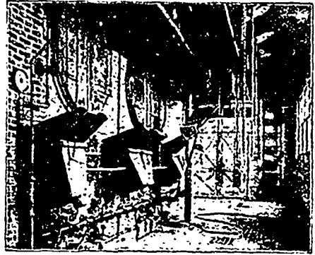
In Power House shown a Pivoted Bucket Conveyor and Traveling Chute for feeding stokers are features.
