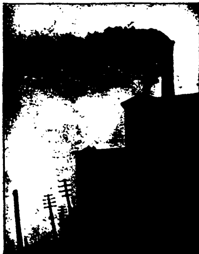
Photograph of a Chimney BEFORE the American Stoker was installed.
