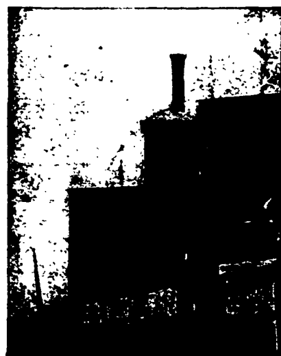
The same THE ... Chimney AFTER American stoker was installed.
