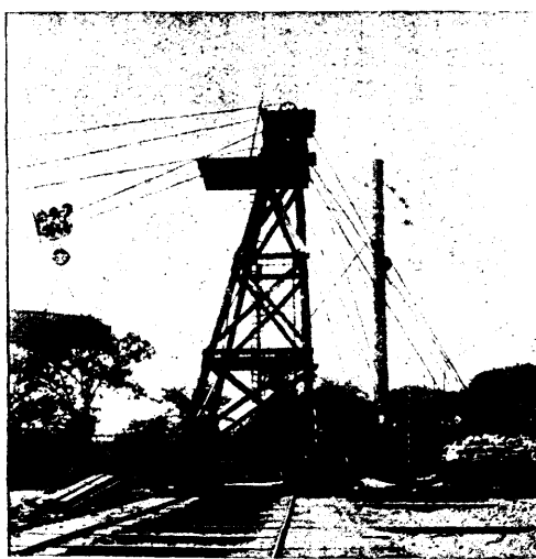
Cable Hoist-Conveyor at St. Paul, Minn.
