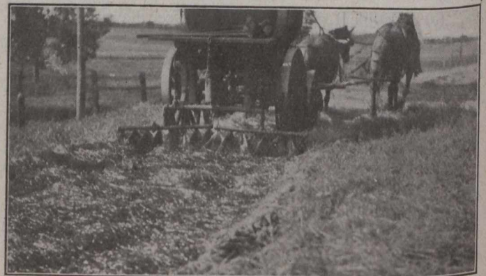
Applying Tar to Straw; First Application
