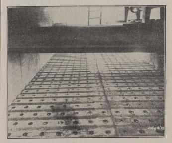
Filter Showing Air Pipes and Cravel, Columbus, Fig. 4. Ohio.
