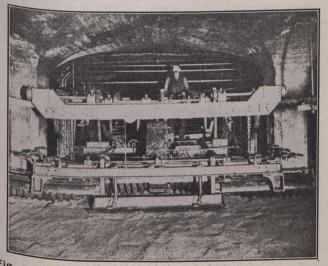
Fig. 3. Filter, Showing Strainer System in Piace, Columbus, Ohio.
