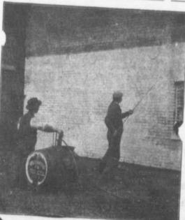
This Photo illustrates the Spramotor (Fig. 4) at work on a barn with two nozzles on the one line of hose. This building was painted in forty minutes after the paint was mixed.
