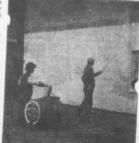
is Photo illustrates the Spramotor (Fig. 4) work on a barn with two nozzles on the e line of hose. This building was painted forty minutes after the paint was mixed.
