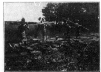
Laying a Corduroy Road
