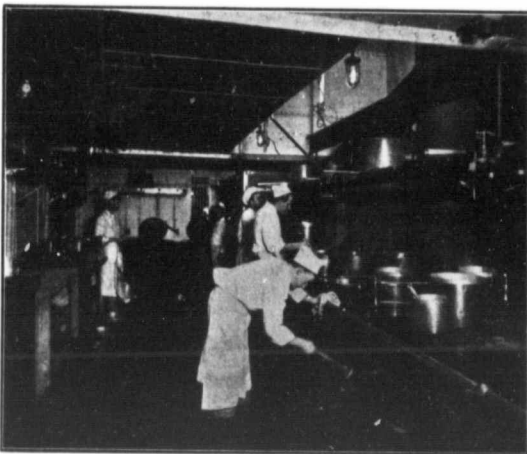
One of the Kitchens. Electricity reigns supreme—Electric Cooking—Electric Washing
