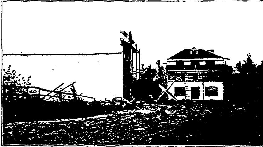
HUDSON'S BAY COMPANY'S STORE AND NEW HOTEL IN COURSE OF CONSTRUCTION
