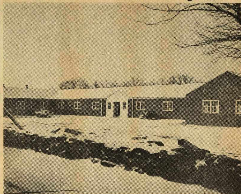
The Shack.—The above building houses the Engineers. Affectionately known as "The Shack", this prefab has served to accommodate the Department of Engineering since it was handed over to the University at the end of the war.
