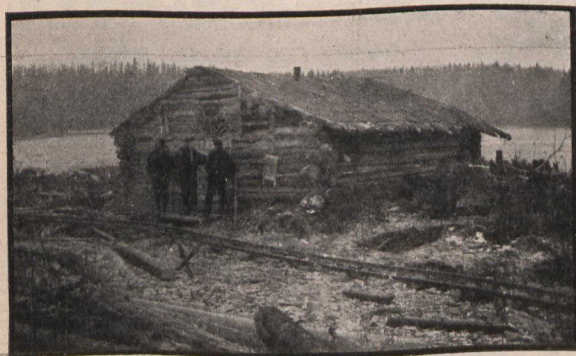
Cache-Keeper's Shack, along the route of the T. & N. O. Railway.
