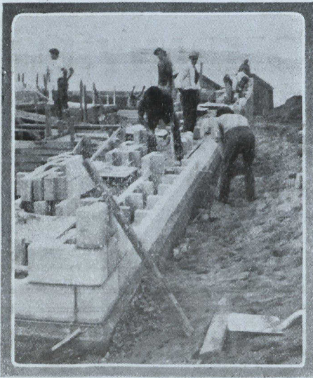
The manner of laying Hydro-stone is here shown. The workman in the right foreground is setting the pre-cast blocks in cement mortar—his helper, working inside the foundation, is placing a row of blocks in readiness for laying.
