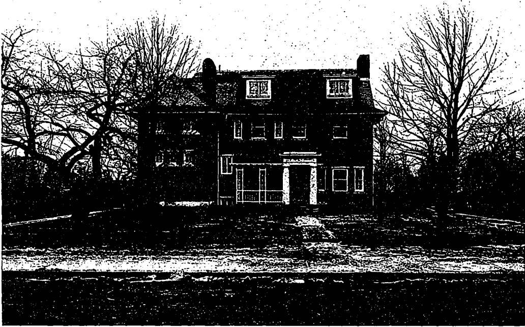
Residence of E. R. Rolph, of the firm of Sproat & Rolph, Architects, on Jackes avenue, Toronto. An interesting Georgian house with walls of ordinary red brick laid in a double stretcher bond, so jointed with false vertical joints of the same colors as to take on the appearance of Roman brick.
