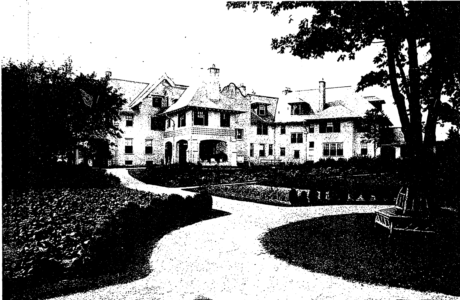
Residence of Wallace H. Rowe, Cobourg, Ont. View showing porte cochere and garden front on north side of house. Rutan & Russell, Architects.
