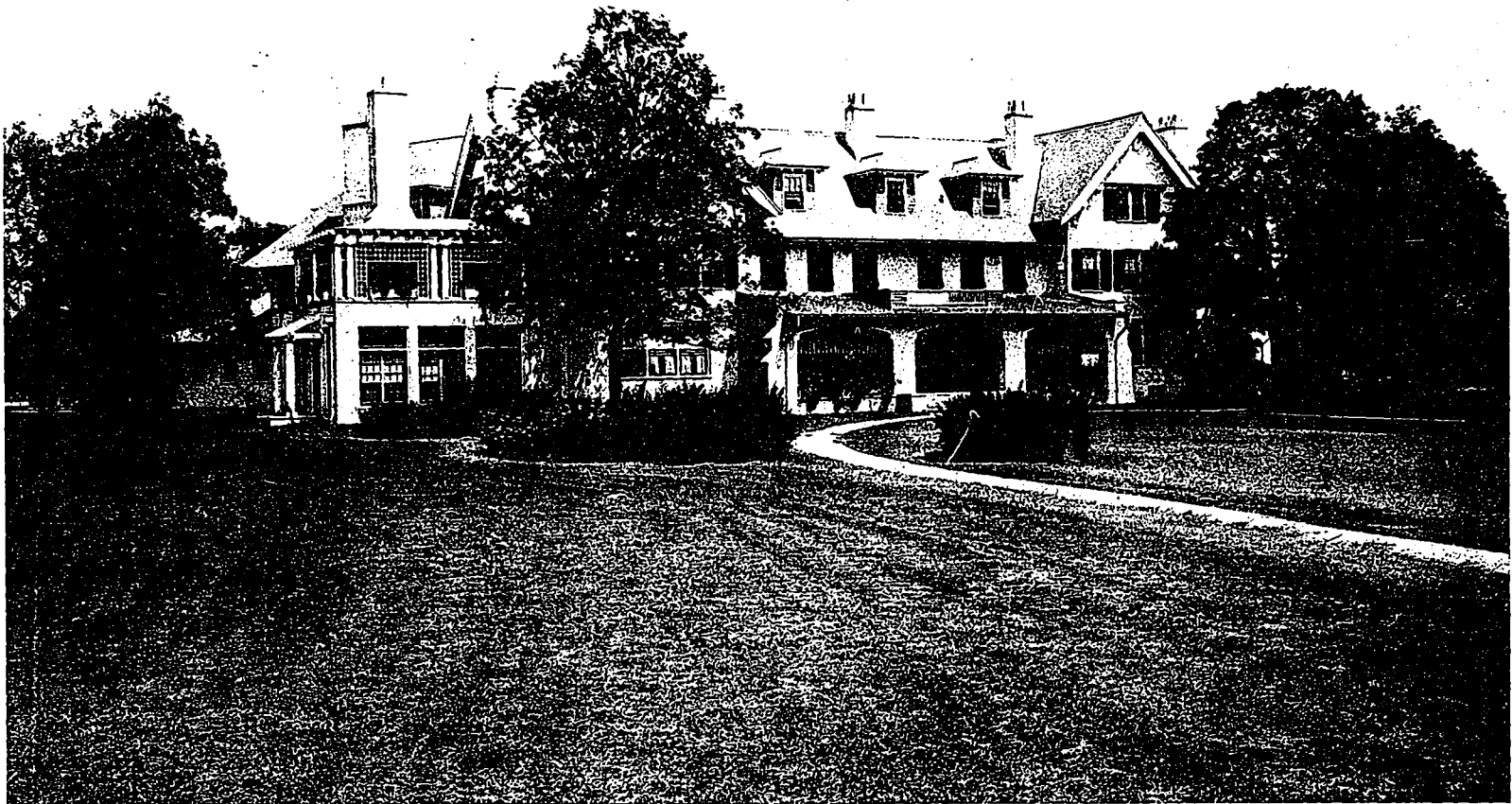
Residence of Wallace H. Rowe, Cobourg, Ont. This house is of fireproof construction throughout, the exterior and interior walls being of brick and tile, and the floors of combination hollow tile and reinforced concrete construction in long spans. The exterior is finished in concrete stucco with a pebble dash surface, cream white in color, and the roof is of tile. Rutan & Russell, Architects.
