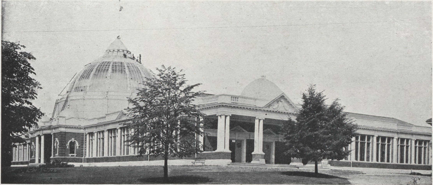
New Horticultural Building, Canadian National Exhibition. George W. Gouinlock, Architect.
