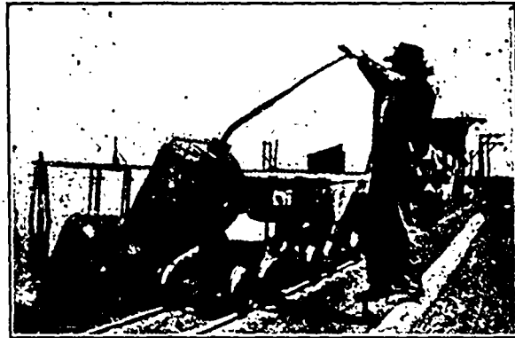
Fig. 2.—Method of Discharging the Slag-Car.
