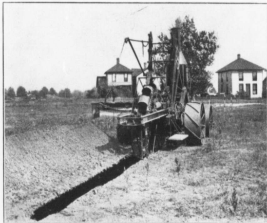
DITCHING MACHINE AT WORK.
