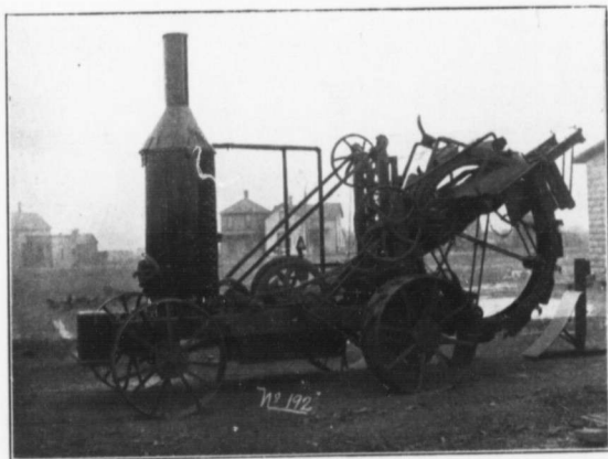
SIDE VIEW OF DITCHING MACHINE.
