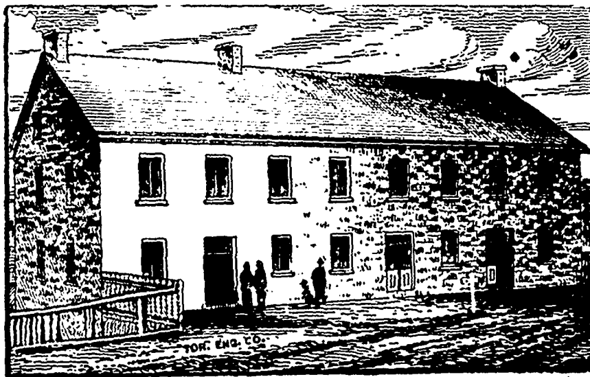
McLAREN & SONS' NEW FLOUR MILL AT ARNPRIOR, ONT.
