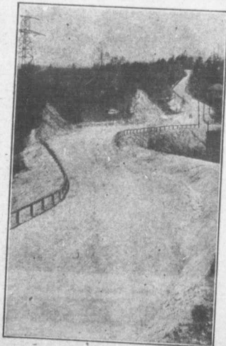
Cuts and Fills Along the Humber, York Co., Ont.
