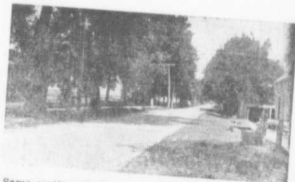
Same section of King Edward Highway, Napierville, Que., after improvement.
