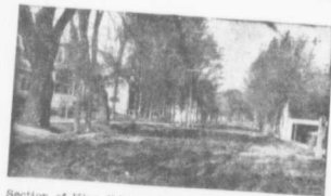
Section of King Edward Highway, Napierville, Que., before improvement.
