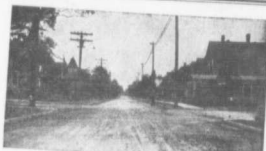
Two-course concrete street, Amherst, N.S., laid in 1914.
