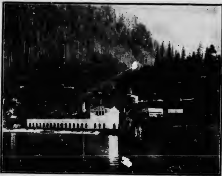
Electric Power Plant
