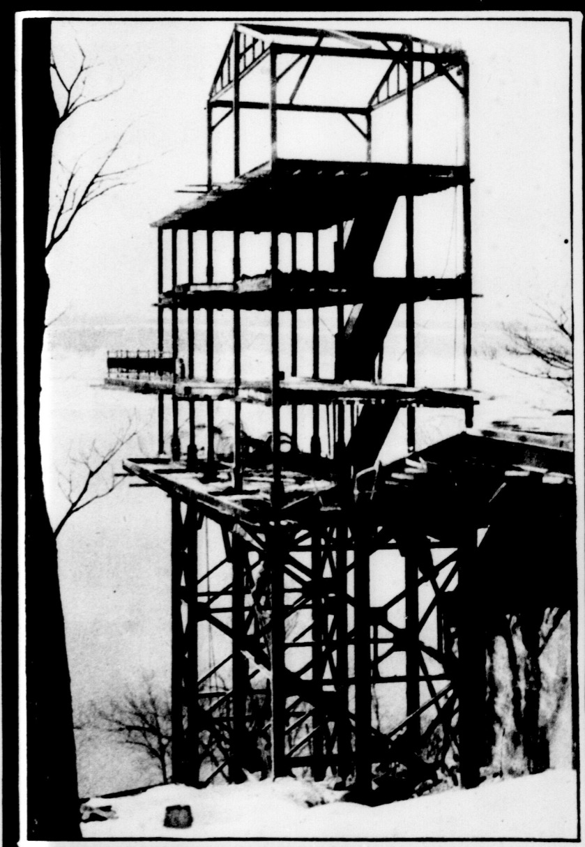
A modern cliff dwelling—a house being built on steel stilts by Cleveland Walcutt of New York on the steep bank of the Hudson river, which will command a wonderful view
