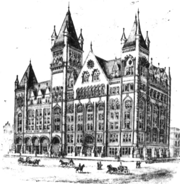
CONFEDERATION LIFE BUILDING.
